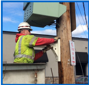
Position the Mounting Bracket at the desired location and mark the top mounting hole on the pole.
