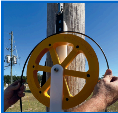
Place cable onto wheel
