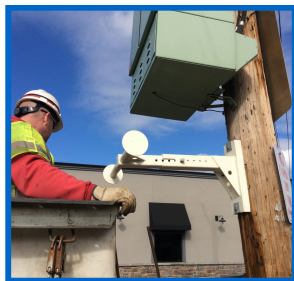
Insert the Support Extension with the Safety Belt Bracket facing upwards.
