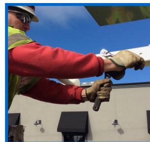
Attach additional fender washer, lock washer, and hex nut onto the bolts and fully tighten using a 5/8" socket and adjustable wrench.
