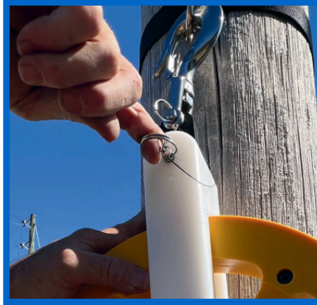
Remove retainer pin
