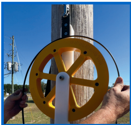
Place cable onto wheel
