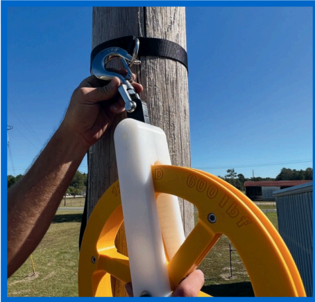
Attach Hi-Roller to existing pole line hardware or pole strap (VPN 59401)
