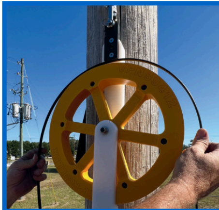
Place cable onto wheel
