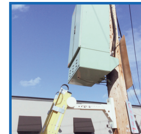
Lean the ladder against the Pole Mounted Ladder Bracket and secure using your company's standard practice.
