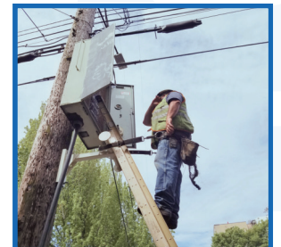
Secure yourself using your safety belt by looping your belt over and through the Safety Belt Bracket.
