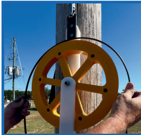
Place cable onto wheel
