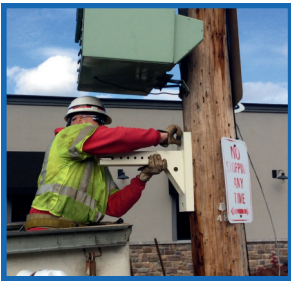
Securely tighten the Mounting Bracket to the pole.
