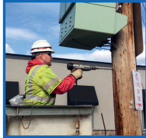
Drill through the pole making sure that there are no obstructions on the opposite side.
