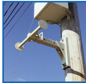
Position the Support Extension to the desired location and line up the holes of the fiber cable to be used in both the Mounting Bracket and the Support Extension.
