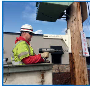
Drill through the bottom mounting hole and insert the pole mounting hardware.
