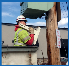
Loosely attach the Mounting Bracket using the appropriate pole mounting hardware.
