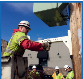
Insert (2) 4" hex head bolts with fender washers into adjusting holes on the side of the Mounting Bracket.
