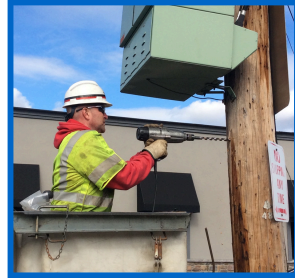
Drill through the pole making sure that there are no obstructions on the opposite side.
