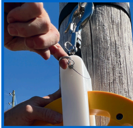
Remove retainer pin
