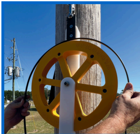
Place cable onto wheel
