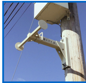
Position the Support Extension to the desired location and line up the holes of the fiber cable to be used in both the Mounting Bracket and the Support Extension.
